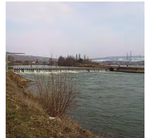
Station de Damery
