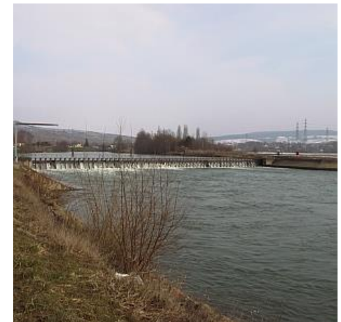
Station de Damery
